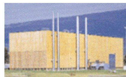
Bi►re in Switzerland, where a 300kW e ORC turbine and wood boiler provide CHP for a barracks and local village.
